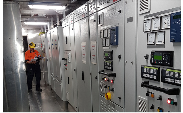
Incat Hull 089: Switchroom termination and commissioning
